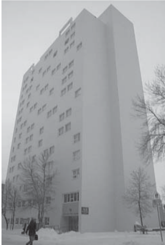
Provincially owned high-rise apartment building located on Kennedy Street in Winnipeg.
