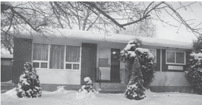
Provincially owned single family residence located in Winnipeg.
