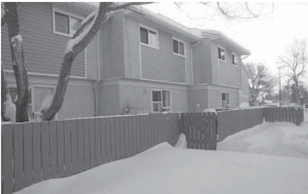
Provincially owned townhouses located in Winnipeg with recently completed exterior retrofits.
